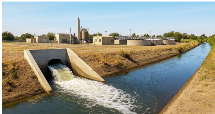
Atwater Municipal Sewage Treatment Plant
