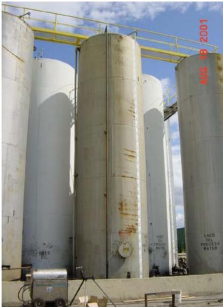
Once the oil has been heated and the water is driven off to less than 1% by volume, the feed waste oil is pumped into the V◇SEP Filter Pack at about 60 psi. The contents of the 20,000 gallon feed tank are processed so that the filtrate is removed from the system and sent to a "Look See" holding tank and then a larger product storage tank. As filtrate is removed by filtration and the reject is sent back to the feed tank, the contents of the feed tank are then
