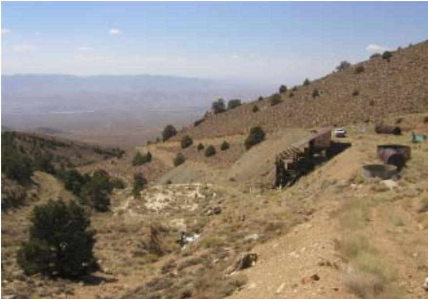
**An abandoned Gold Mine located in Nevada. The picture shows the remnants of the headframe used for the crushing operation. Also shown are the tanks used for processing of the slurried gold ore. The tailings pond is located down below the headframe**
