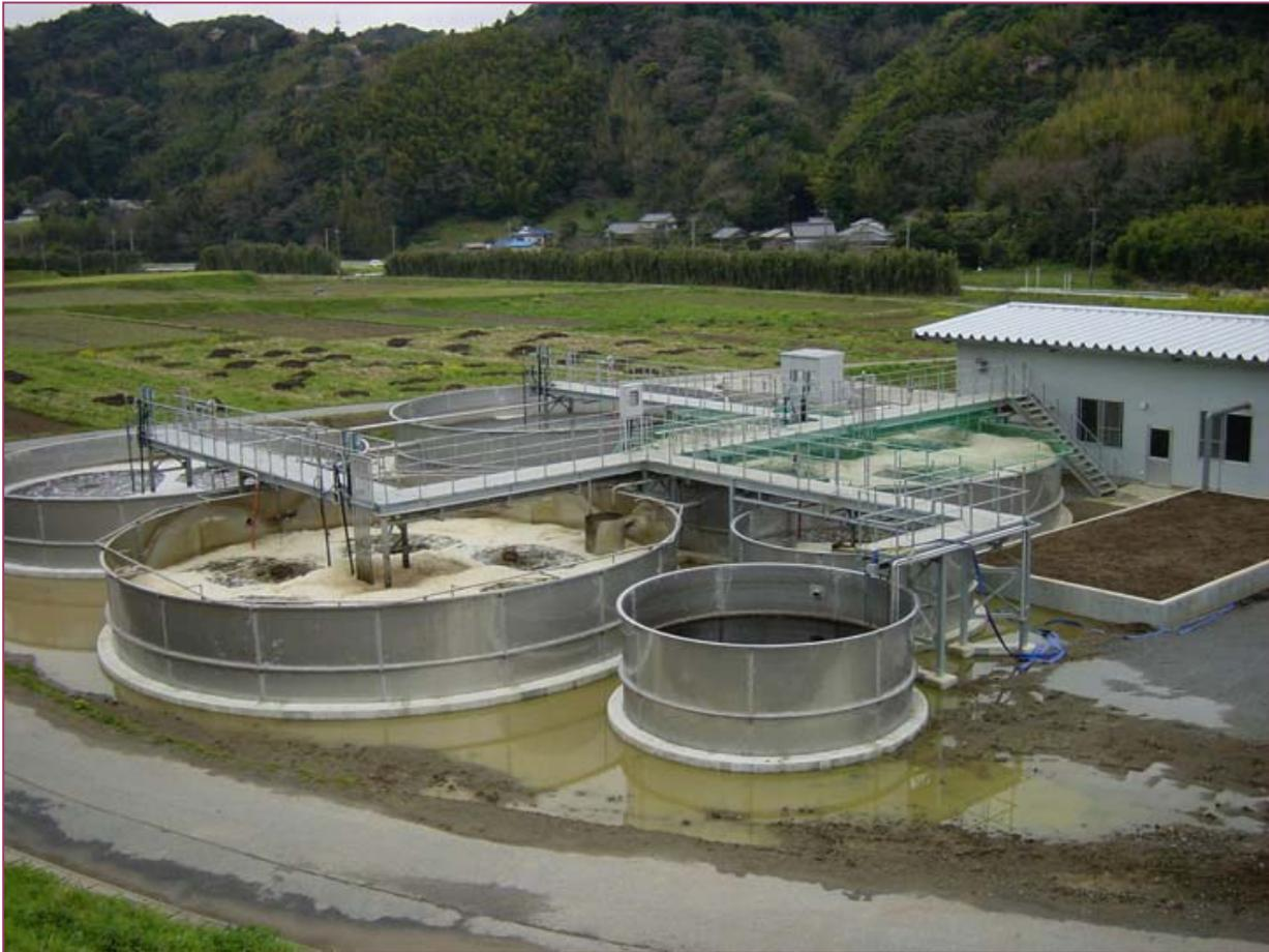
**Typical Outdoor Aerobic Digester (Japan)**
