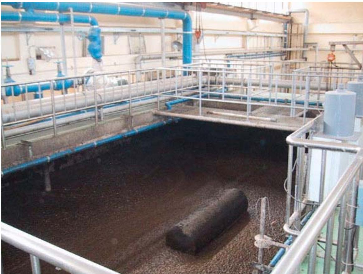
Sequencing Batch Reactor (Feed to V $\diamond$ SEP)
